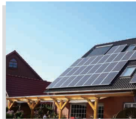
Solar System Set P11 - 13
