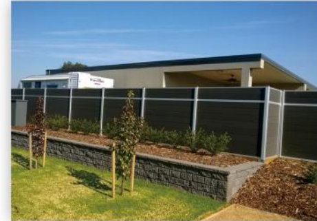
1. Superhigh fence installation
