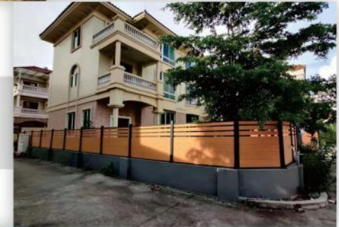
2. Irregular corner fence installation
